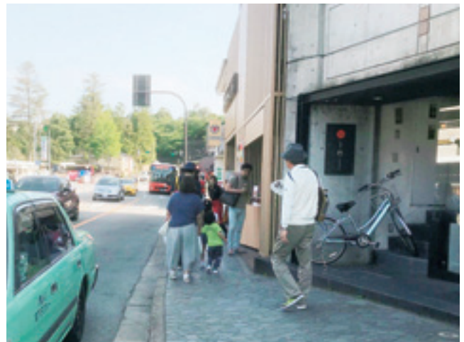
写真-2 歩道が狭隘
